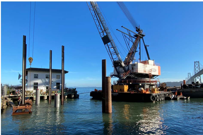
Fireboat Station 35 Pile Driving at Pier 22½
