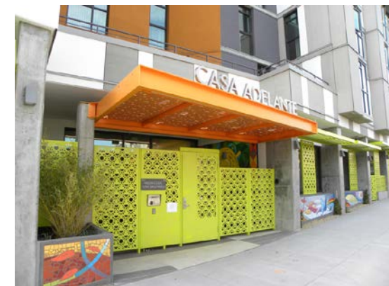
Casa Adelante - 1296 Shotwell construction complete and fully-occupied
